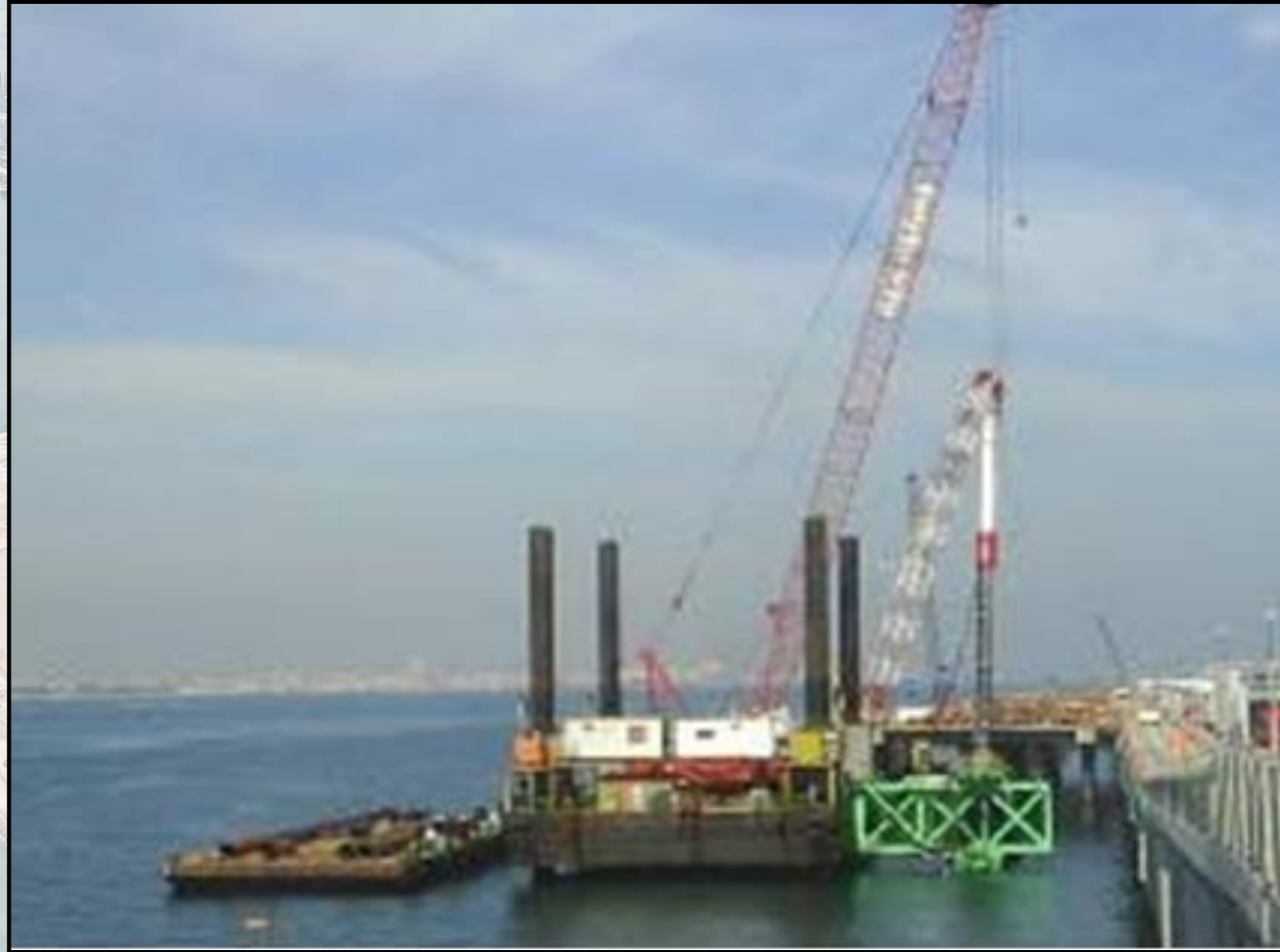
< Placing Pile and Installation of Hammer >
