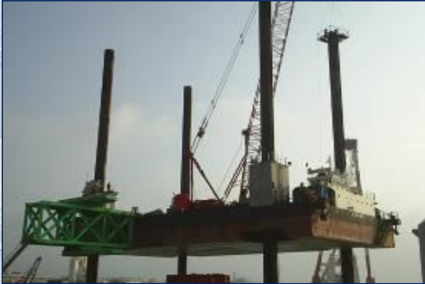
< Setting of Jack-up Barge >
