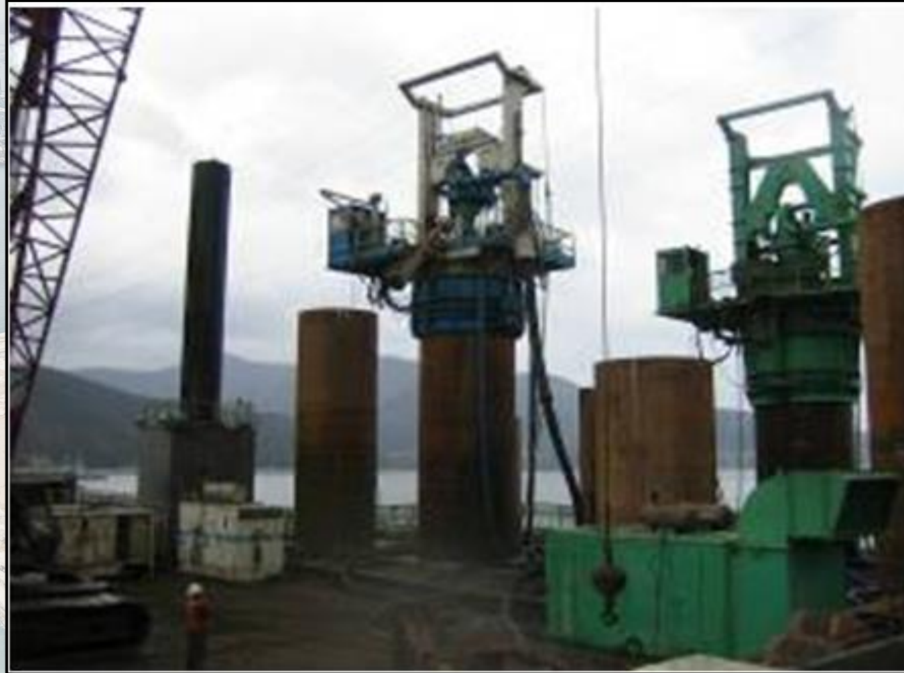
< Pile Driving with Drilling (RCD) >
