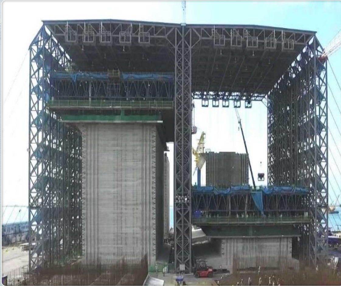
< Wall Casting by Slipform >
