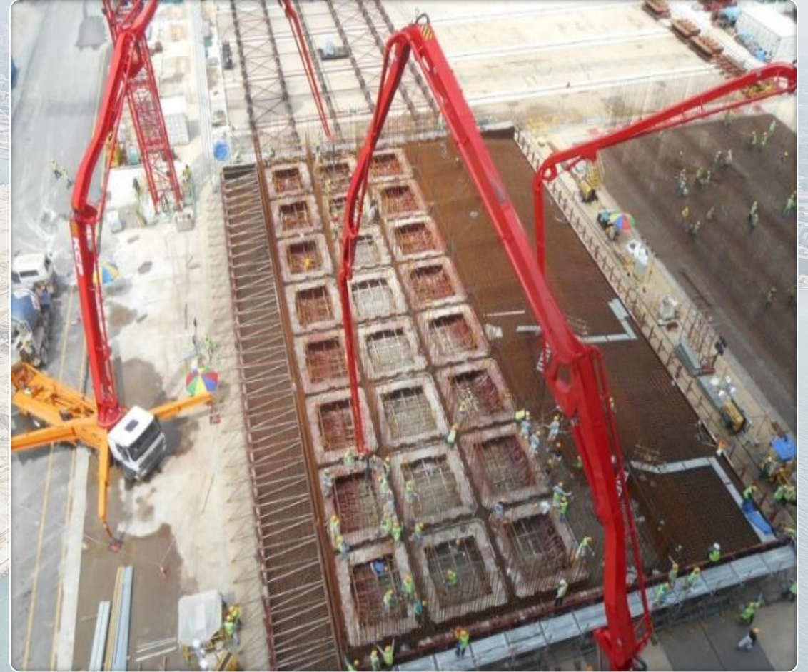
< Base Slab Casting >
